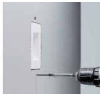
Screw the spot together with the plasterboard
