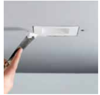
Plaster spot and wall and paint with desired color
