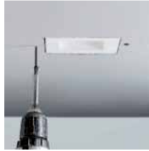
Screw the spot together with the plasterboard
