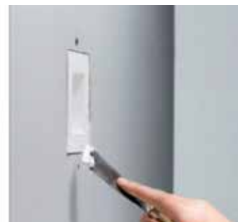
Plaster spot and wall and paint with desired color
