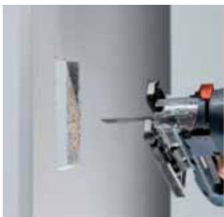
Take measurements and cut the plasterboard
