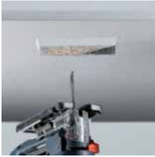
Take measurements and cut the plasterboard
